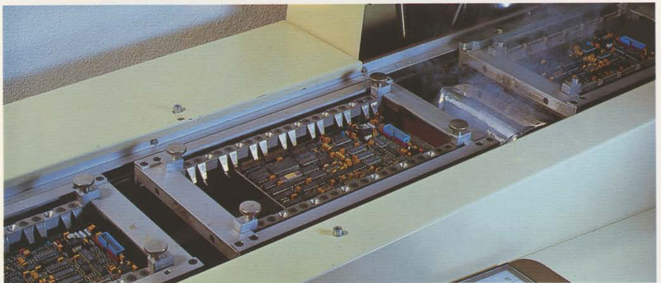
The automatic wave flow solder system can handle up to 3,000 boards per month
